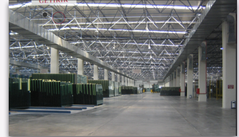
Trakya Glass Factory Project Türkiye | 2023
